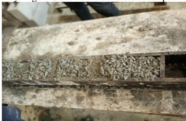
Figure 7: Casting and Vibration of concrete moulds.
