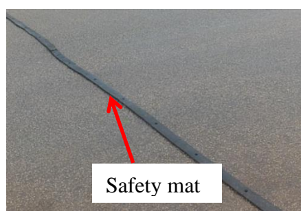
(b) Fibre cable covered with safety mat
