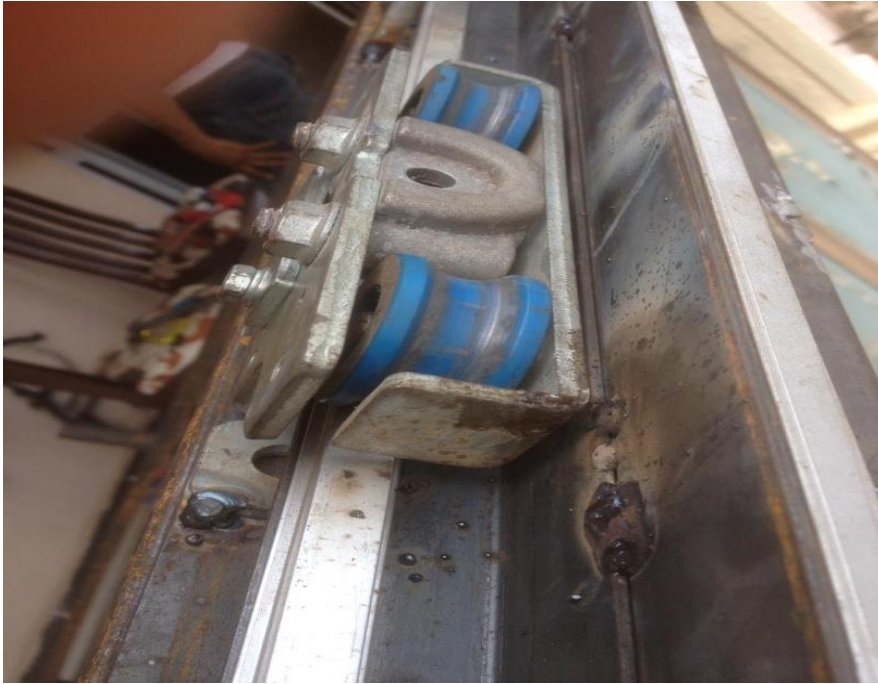
Figure 6. The main rollers of the sliding door
