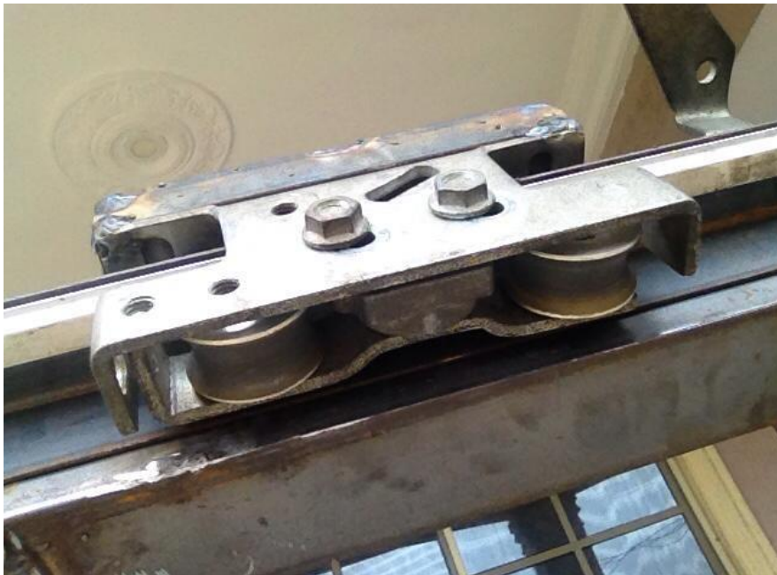
Figure 7. The supportive rollers of the sliding door
