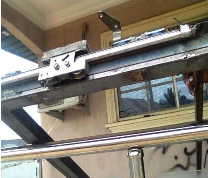
Figure 8. A pictorial view of both the main rollers and the supportive rollers
