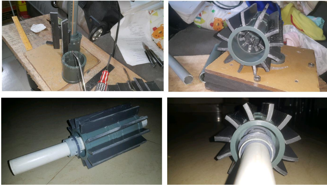
Figure 10: Construction of Component Parts of Water-Ring Pump
