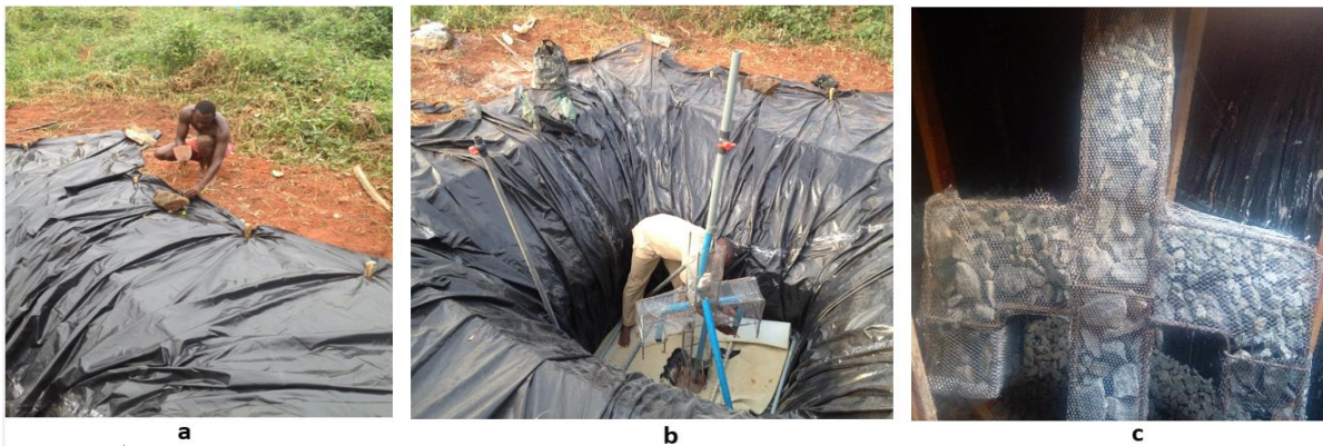
Figure 7: Installation of HDPE Liner, leachate collection pipes and gas extraction well
