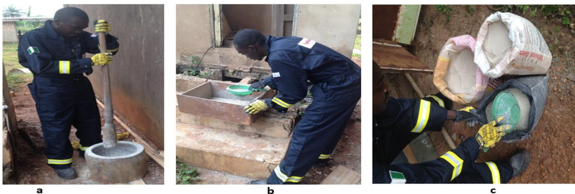
Figure 5: Processing of clay for the landfill basal liner
